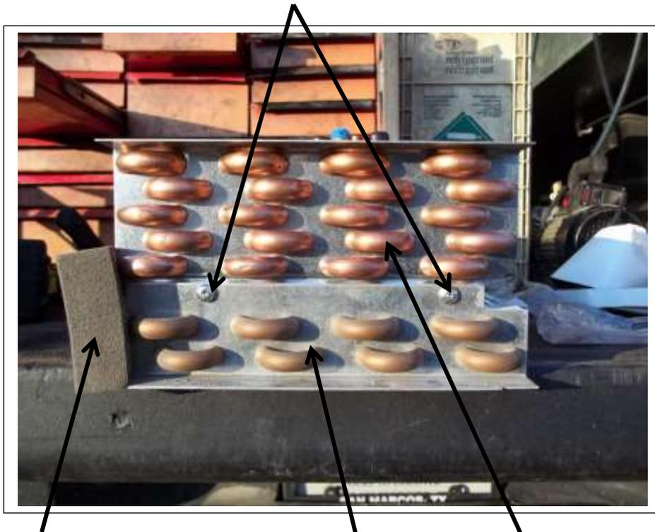
Trim back the foam on top of the heater coil so it butts up tight to the foam on the top of the evaporator coil. (the evaporator foam is not shown in this early picture.)
