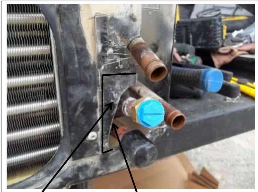
Cut out this are of this metal plate to accommodate the AC lines.
