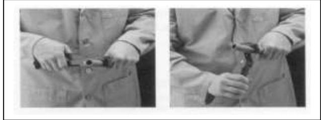
Step 2. Install two proper-sized clips onto the cut end of the hose. Orientation of the clips does not affect the performance of the connection. However, for ease of assembly, both clips should have the same orientation. NOTE: Failure to slide the clips over the hose at this time will require the clips to be stretched over the hose or fitting later. This may permanently damage the clip.
