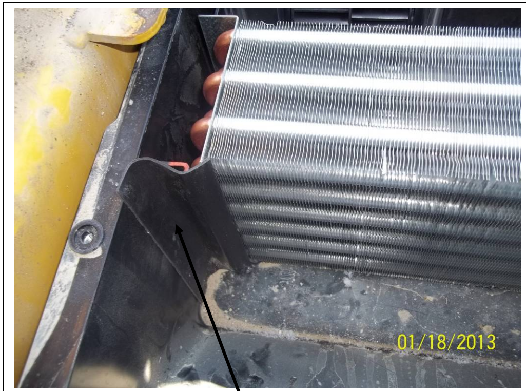
Use self stick tape to seal evap coil into box.
