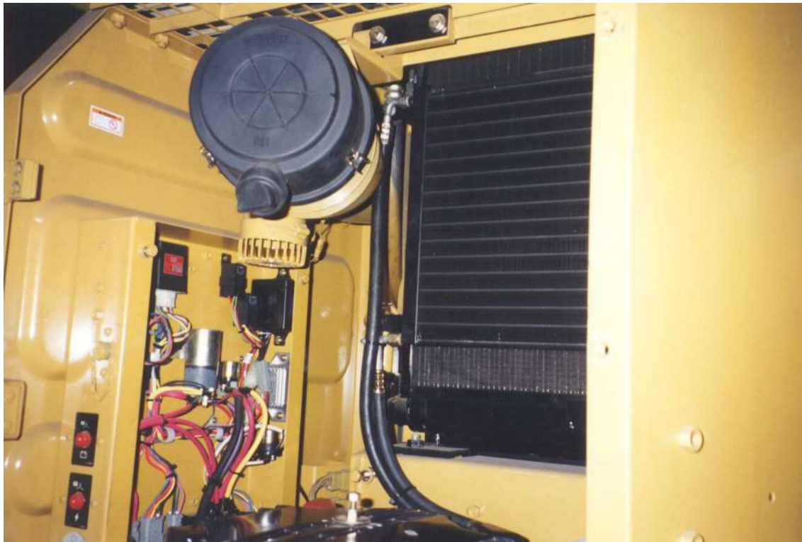
Fitting side of condenser in place.
