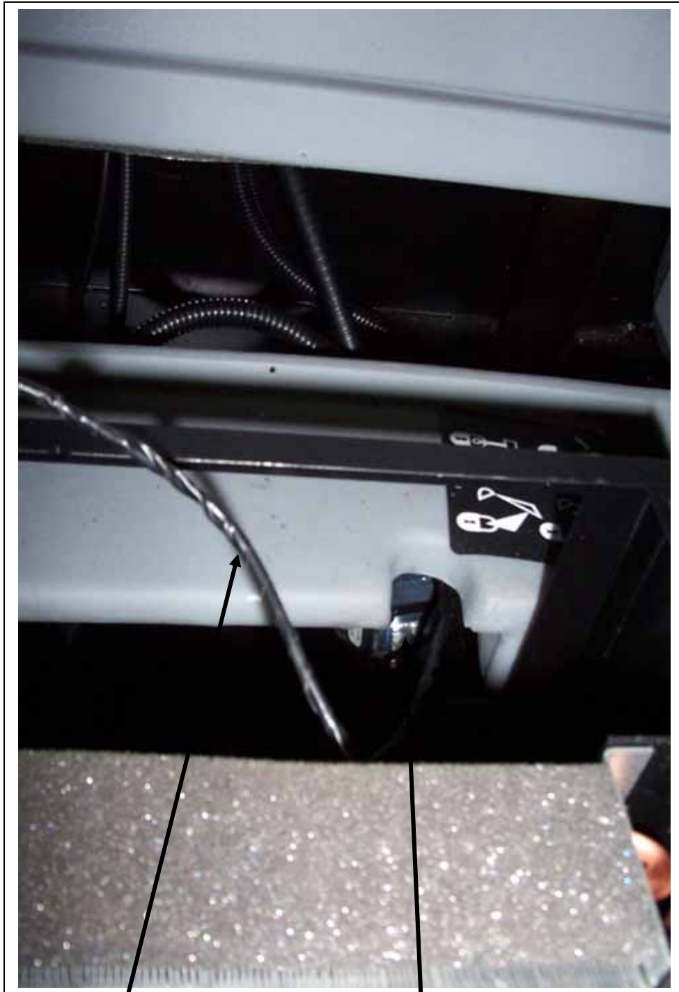
Thermostat probe run before AC coil installed
