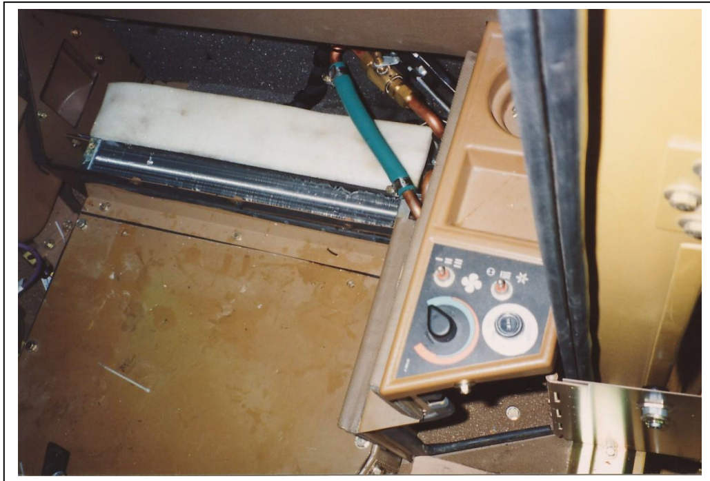
Thermostat location. Hole must be drilled.
