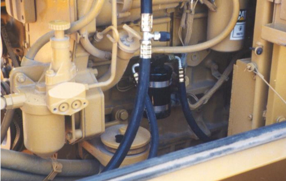
Drier in place.
