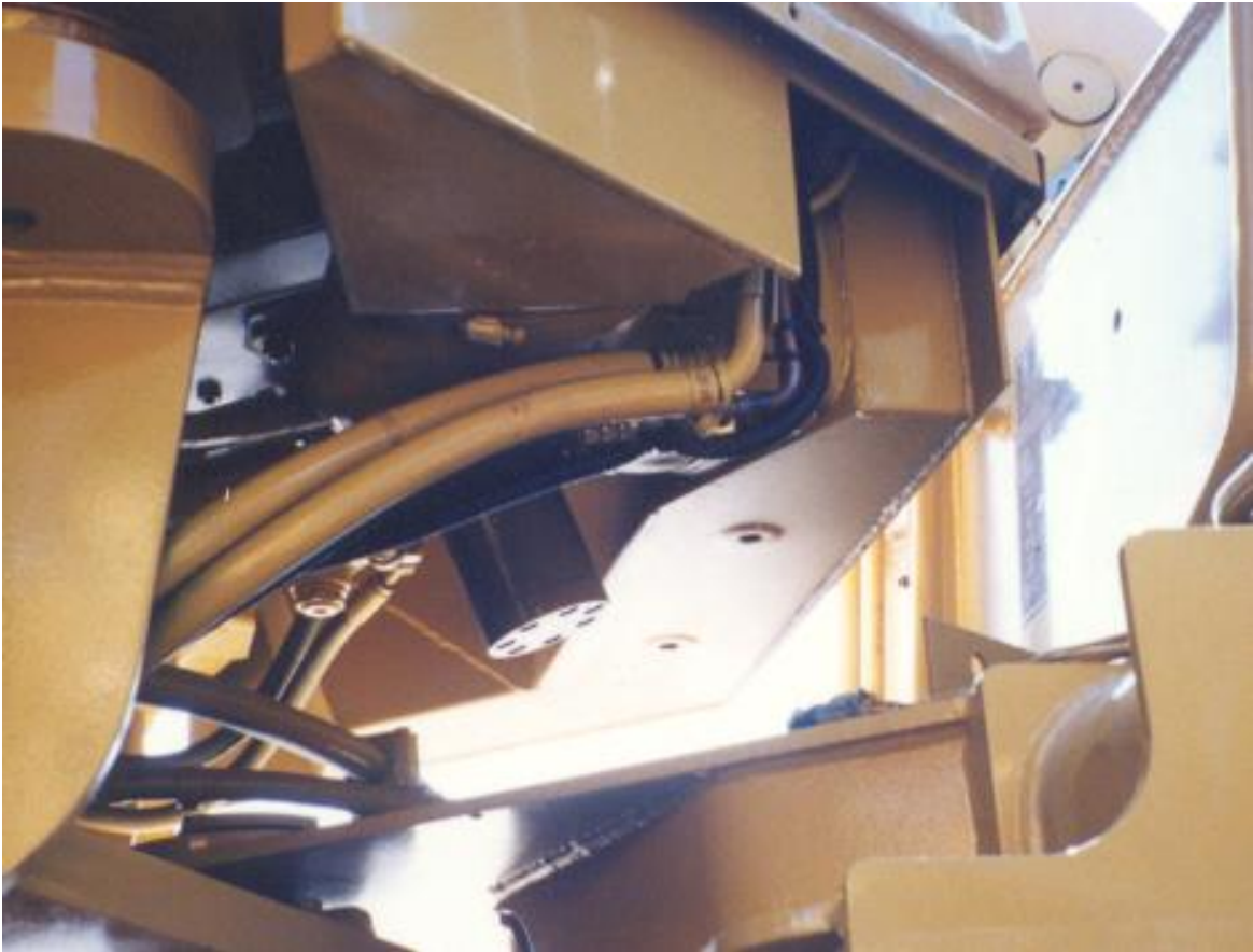
Underside of cab showing hoses to evaporator.
